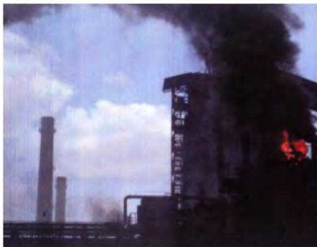
Figure 1 A Cairo, Egypt coke and chemical plant
